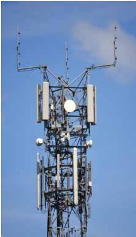
**Figure 4:** Cell site with multiple operator's antenna configurations for 2G and 3G
