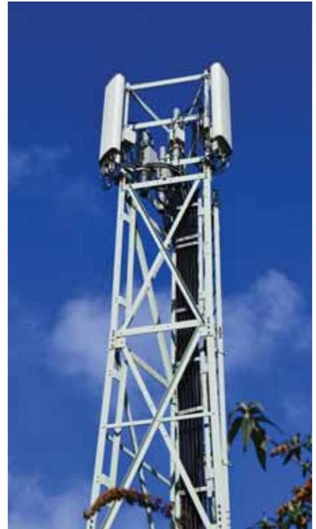
**Figure 5:** Multi-band cell site with 6-port cross-polarised antennas
